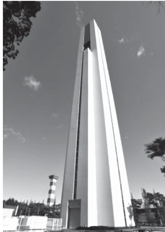
Fig. 22—New Elevator Research Tower. The 213-m elevator research tower is located at Hitachi's Mito Works, and was built with the aim of representing Hitachi as global No. 1 in elevators.
