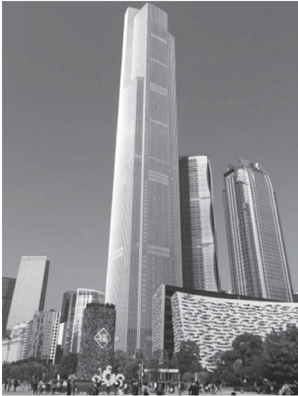
Fig. 24—Guangzhou CTF Finance Centre. The photo shows the building under construction in Guangzhou, China. Hitachi's 1,200-m/min elevator was already operating at the time.
