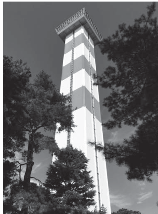
Fig. 1—Old Research Tower. The old research tower is 90 m tall and was completed in 1967. It is still used for elevator development.
