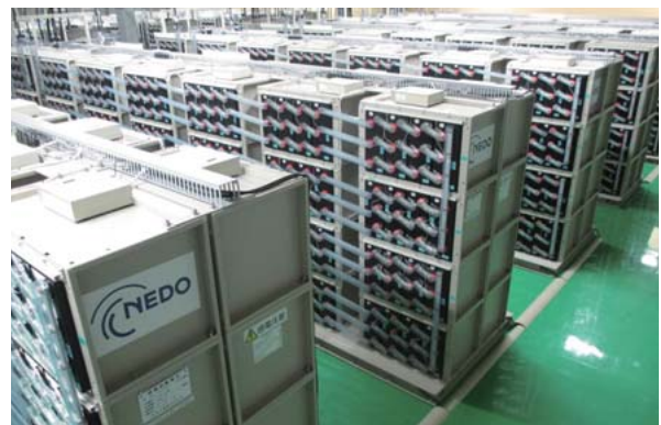
3 New lead storage battery equipment installed on Izu Oshima Island
