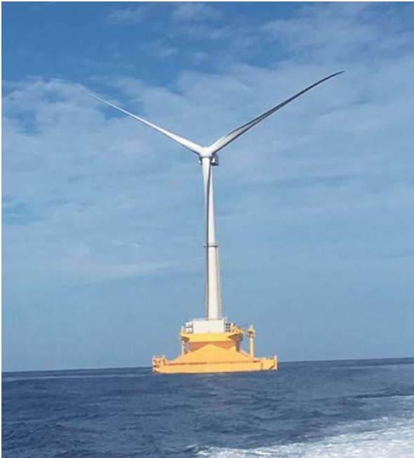
4 5 MW down-wind floating wind turbine (photograph courtesy of Fukushima Offshore Wind Consortium)
