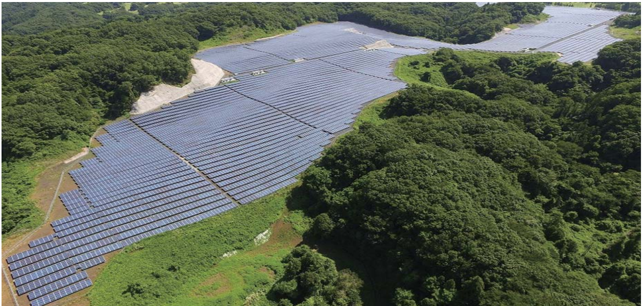
6 Arrangement of solar battery panels through pile foundations that utilize the topography of a golf course
