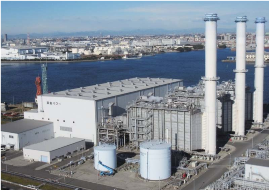
1 Panoramic view of the Ohgishima Power Station
