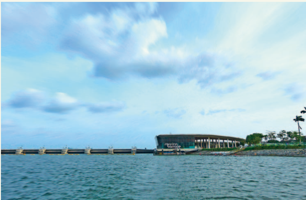
Dam Facility “Marina Barrage” at Marina Channel Estuary
